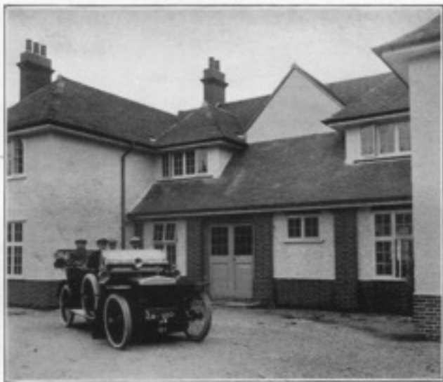
Alderman Paul at the Sanatorium Main Entrance.
