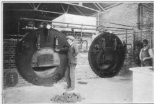
The Boiler House.
