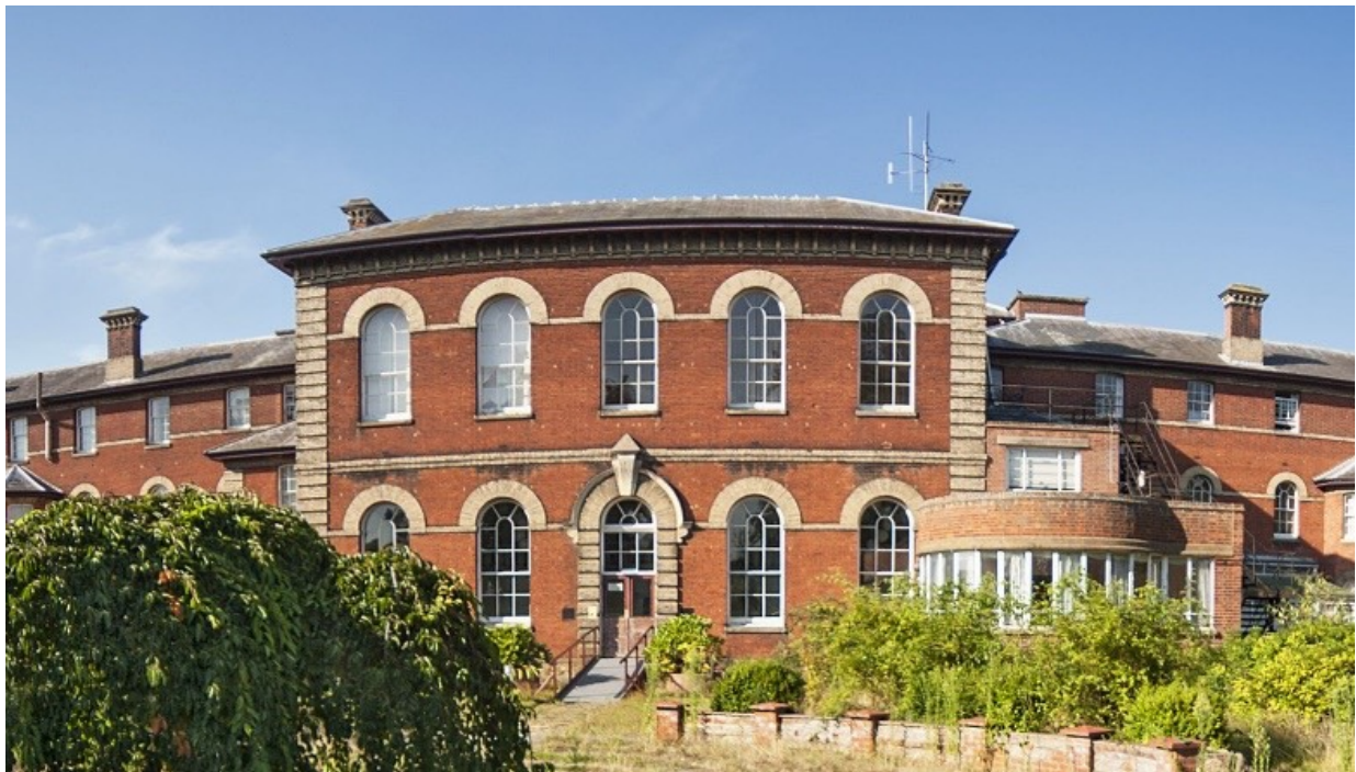
St Clement's Hospital designed by William Parkes Ribbans (countyasylums.co.uk)
